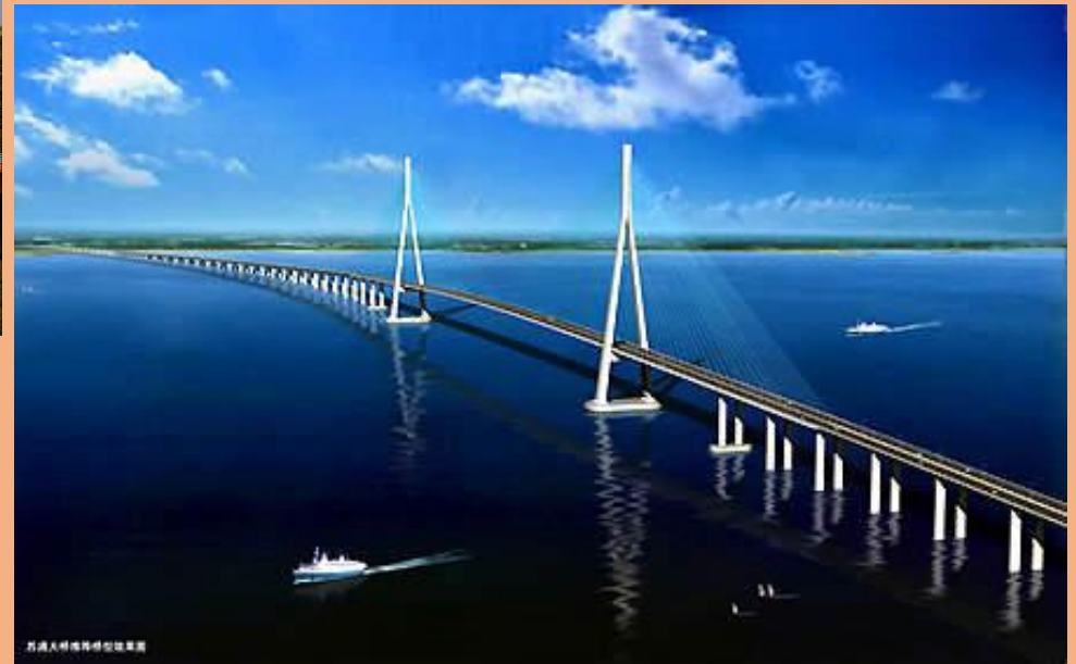
Sutong Bridge – span 1,088m. Built 2008
